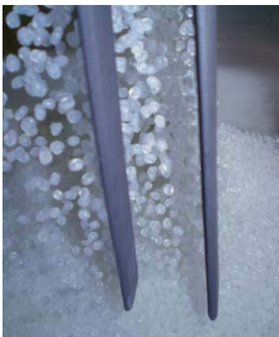
Level switch in a plastic pellet silo
