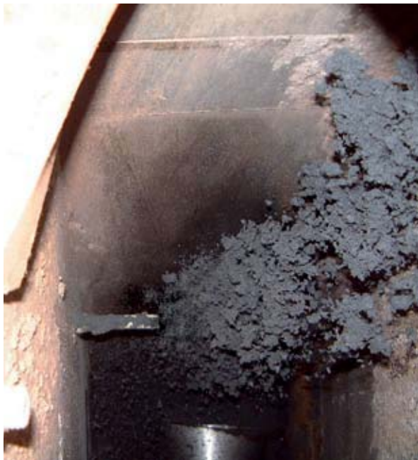
Continuous filling with build-up on probe
